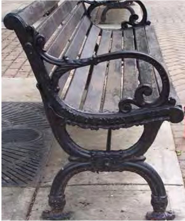
sidewalk,. Opposite the Alley benches face toward the street. All benches are cast iron framing with wood slats. Wood slats in disrepair need to be painted or replaced. If replaced, composite materials should be considered to reduce maintenance.
