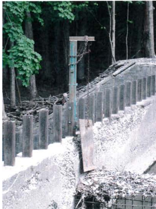
Photograph No. 12: Steel plate used to close outlet of drop-inlet structure.
