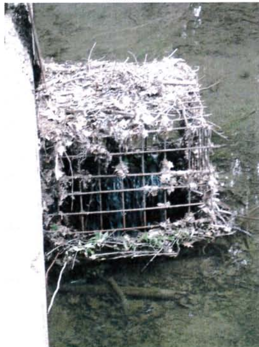
Photograph No. 10: Drop-inlet structure.
