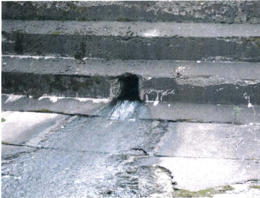
Photograph No. 11: Outlet from drop-inlet structure.
