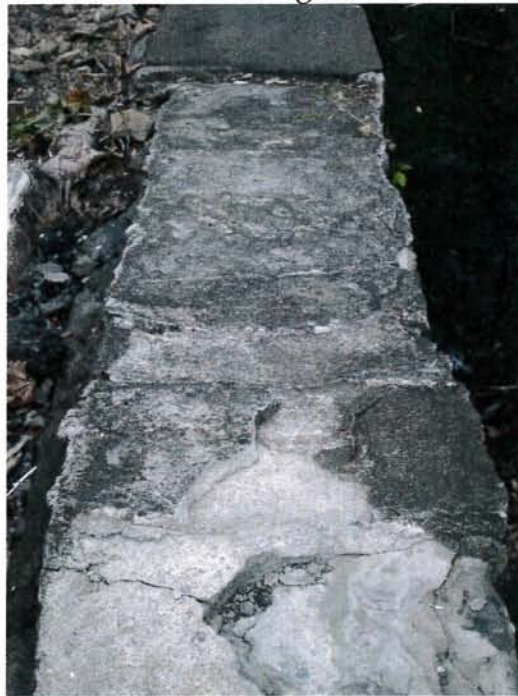
Photograph No. 14: Training wall-embankment interface.
