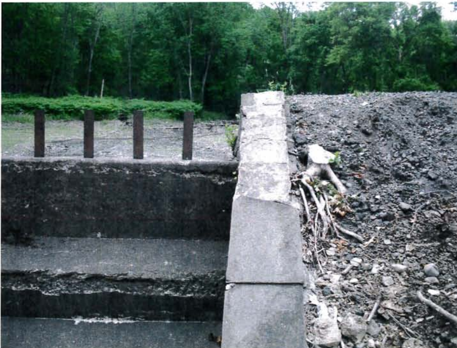
Photograph No. 4: Tree stump and associated root mass on downstream slope of left closure embankment.
