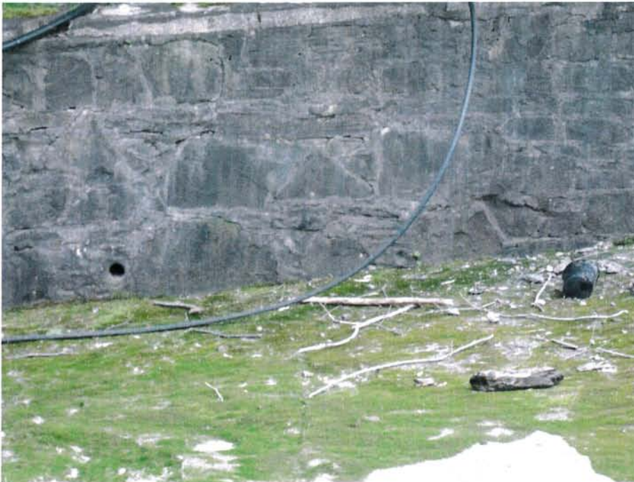
Photograph No. 2: Drain pipe along left abutment wall.
