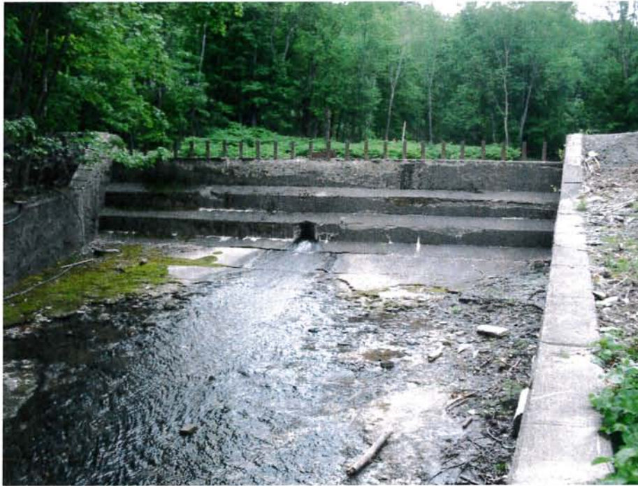
Photograph No. 1: Silver Creek Detention Basin Dam.
