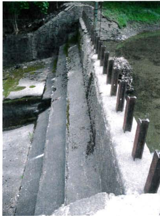
Photograph No. 7: Concrete spillway of Silver Creek Detention Basin Dam.
