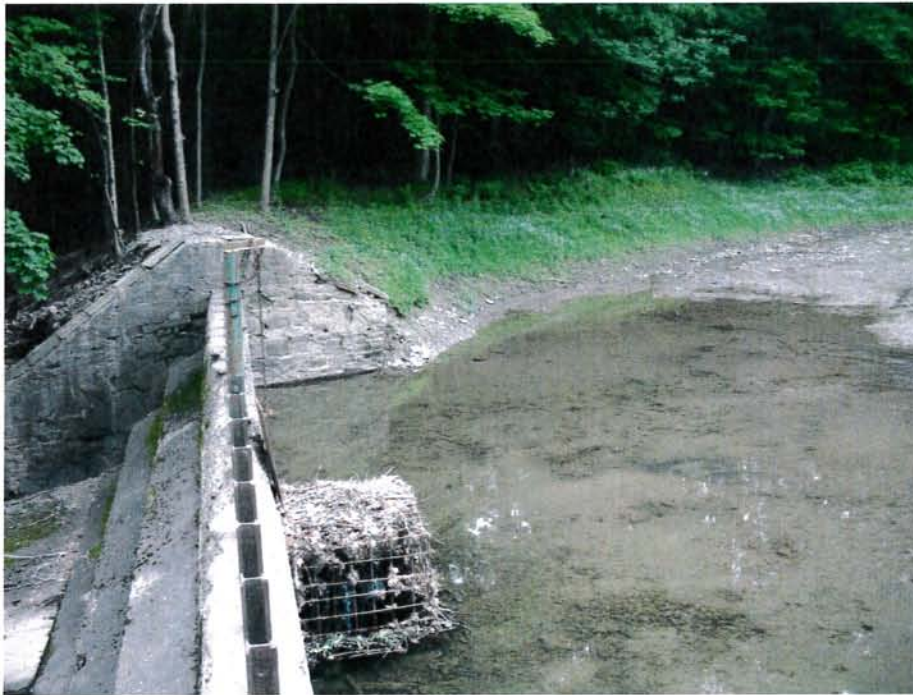
Photograph No. 3: Upstream slope of right closure embankment.
