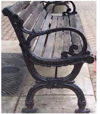
sidewalk,. Opposite the Alley benches face toward the street. All benches are cast iron framing with wood slats. Wood slates in disrepair need to be painted or replaced. If replaced, composite materials should be considered to reduce maintenance.
