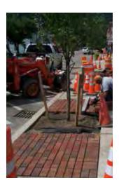
PAVEMENT REPLACEMENT w/ STRUCTURAL SOILS & PERVIOUS PAVERS (Montour Falls, New York) provide 100% surface permeability.
