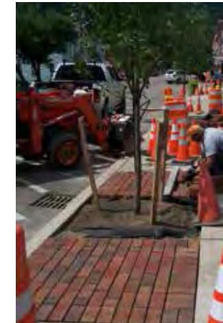
**PAVEMENT REPLACEMENT w/ STRUCTURAL SOILS & PERVIOUS PAVERS** (*Montour Falls, New York*)
