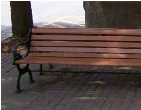
sidewalk,. Opposite the Alley benches face toward the street. All benches are cast iron framing with wood slats. Wood slates in disrepair need to be painted or replaced. If replaced, composite materials should be considered to reduce maintenance.
